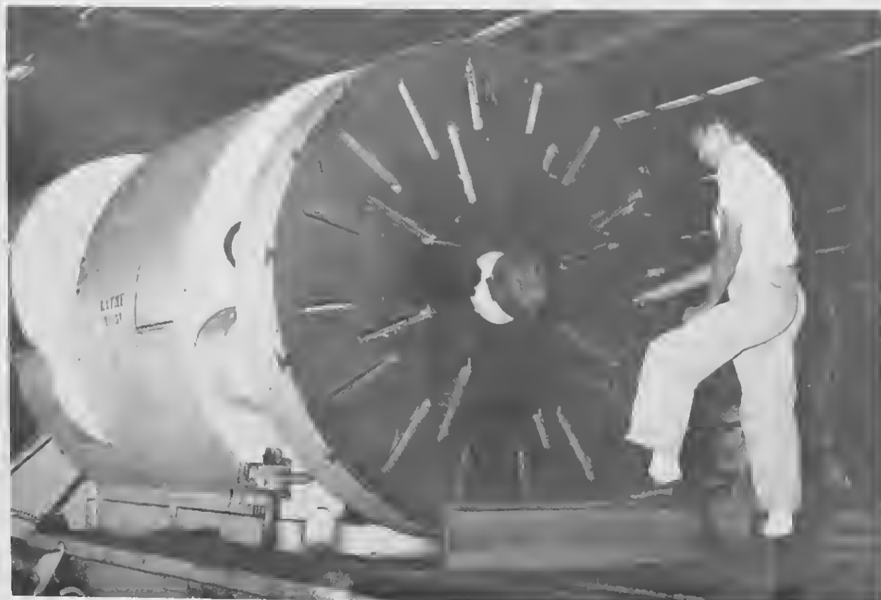
AN AWESOME sight in the Machine Shop is this giant engine lathe which can handle work pieces up to six and one-half feet in diameter. It is used principally to turn down powerhouse turbine rotors. Operator is I. Lampe.
